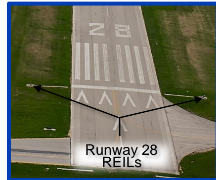
Photo Source: ODOT
